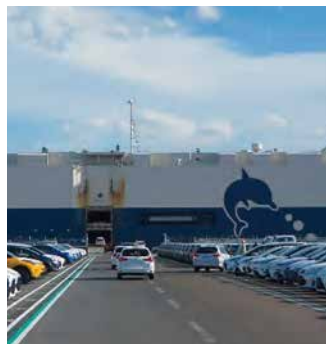
Port of Sendai-Shiogama (Sendai Port District) Raijin Wharf
