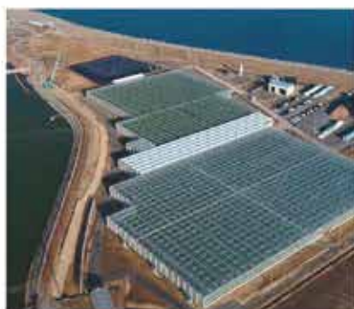
"Next-generation" facility for bell pepper and tomato production
