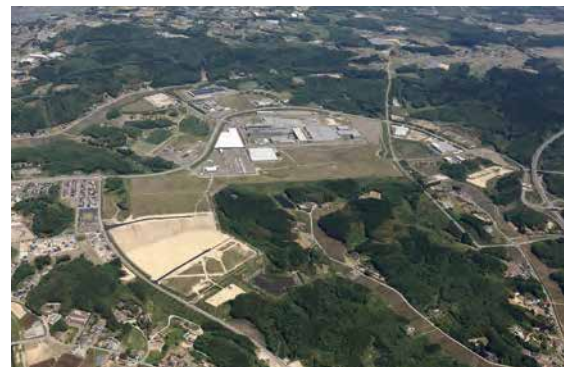
Northern Sendai No.2 Core Industrial Park (Ohira Village)
