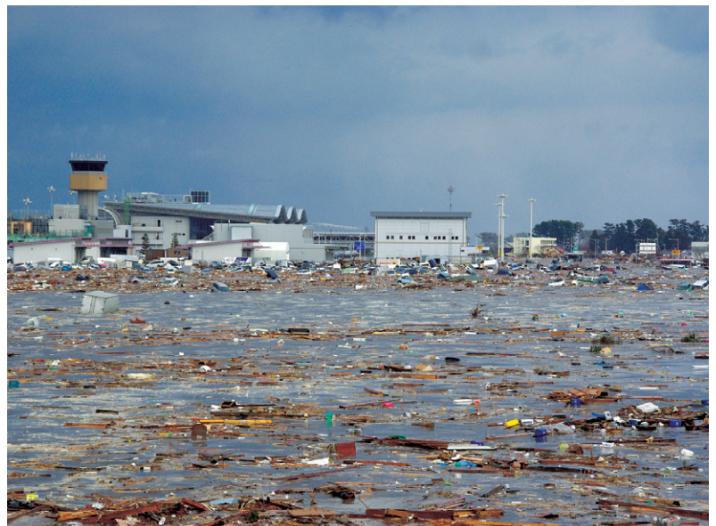
Sendai Airport covered with debris (Photo: 2 nd Regional Japan Coast Guard Headquarters)
