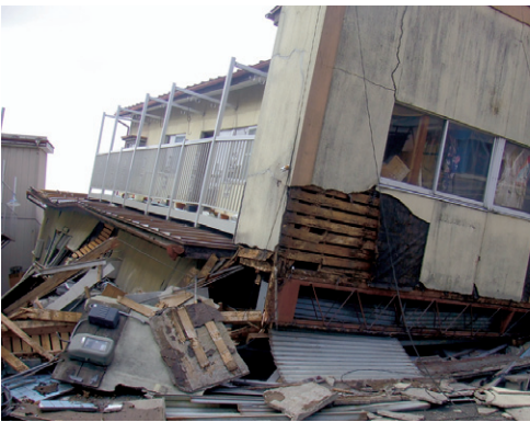
March 18: Collapsed building in Hasama-cho, Tome City
