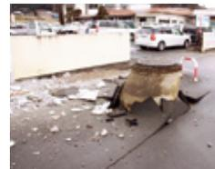
The earthquake caused the liquefaction of the ground and the ejection of manholes across the district.
