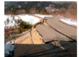
The earthquake caused serious damage to the road, including the collapse of slopes on the prefectural road connecting Shiroishi City with Shichikashuku Town.
