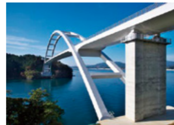
Photo: Kesenuma Oshima Bridge
