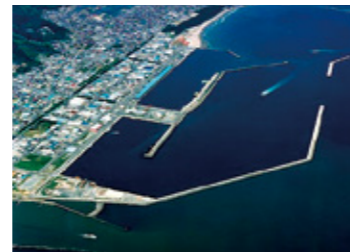
Photo: Ishinomaki Fishing Port under restoration work
