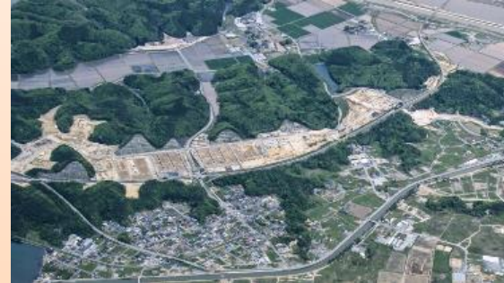
Construction carried out in hills of northern Nobiru (Higashi-Matsushima City)
