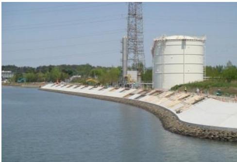
State of reconstruction work on Sunaoshi River (Tagajo City)
