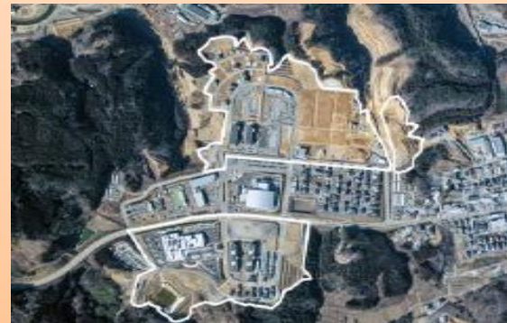
Construction carried out in Shizugawa-Higashi area (Minamisanriku Town)
