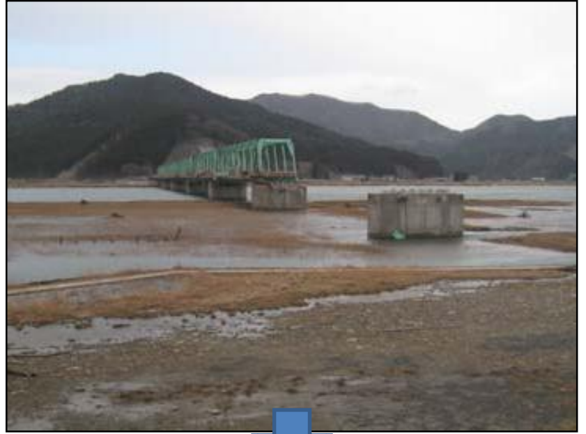
Shin Kitakami Ohashi Bridge (Ishinomaki City)
