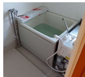
[浴室に浴槽・風呂釜を整備]
