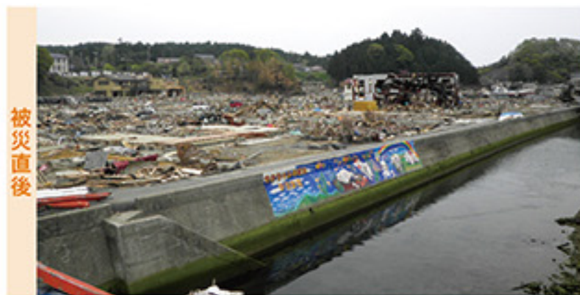
被災直後 Immediately after the disaster
